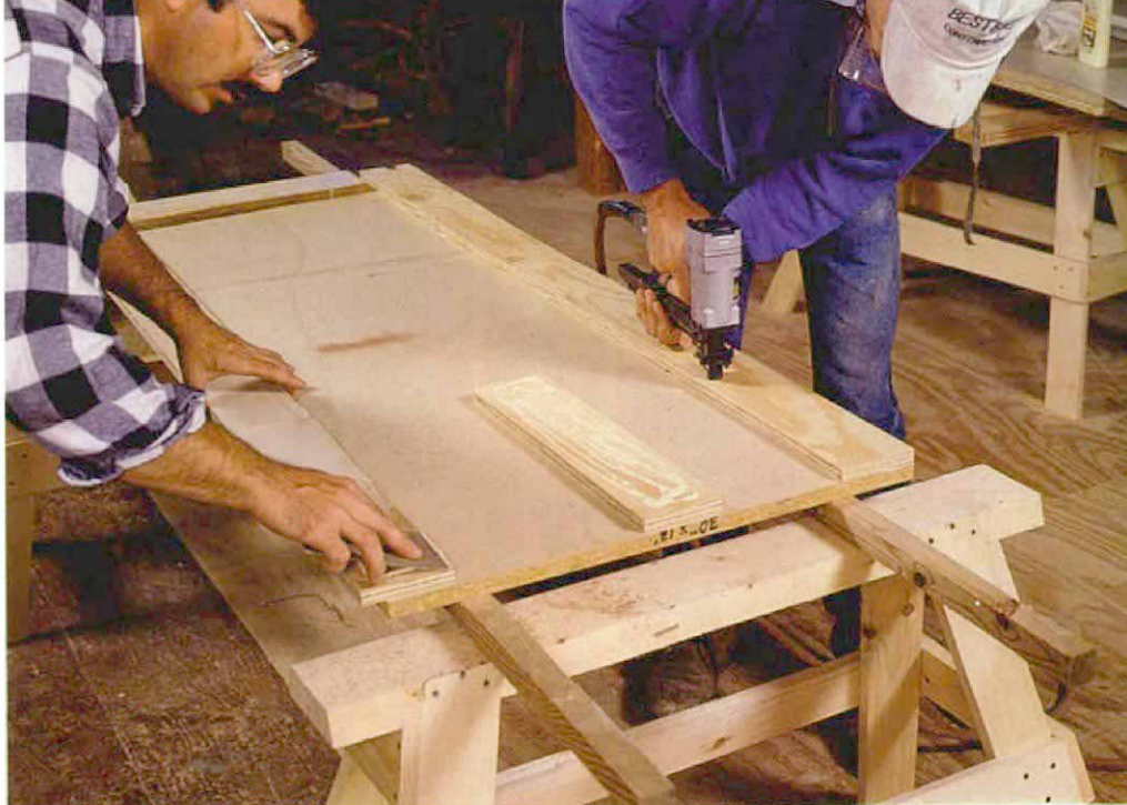
Beefing up the substrate. With its flat, uniform surface, high-density particleboard works best as a substrate for laminate. But gluing and stapling strips of plywood under the edges (and the seams) of the particleboard makes a stronger countertop.
